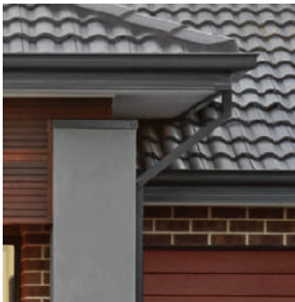
COLORBOND DOWNPIPES, FASCIA & GUTTER
