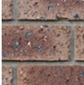
NATURAL ROLLED MORTAR JOINTS
