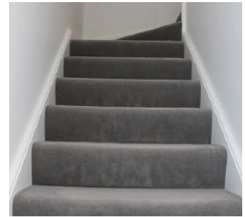
MDF CARPET AND CLOSED STRINGERS TO STAIRCASE
